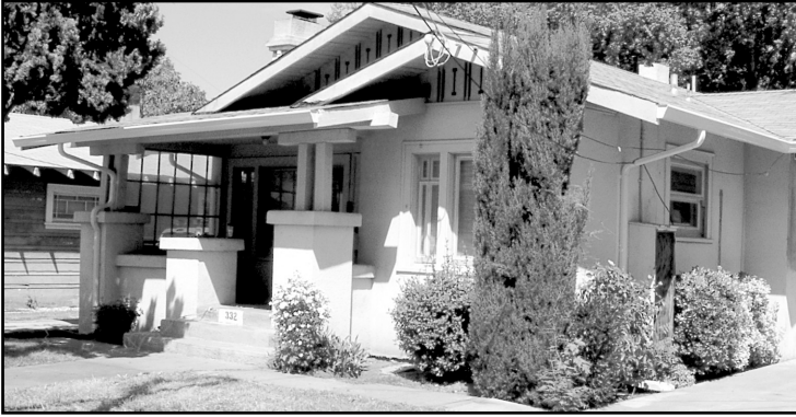
In the middle of a restoration
